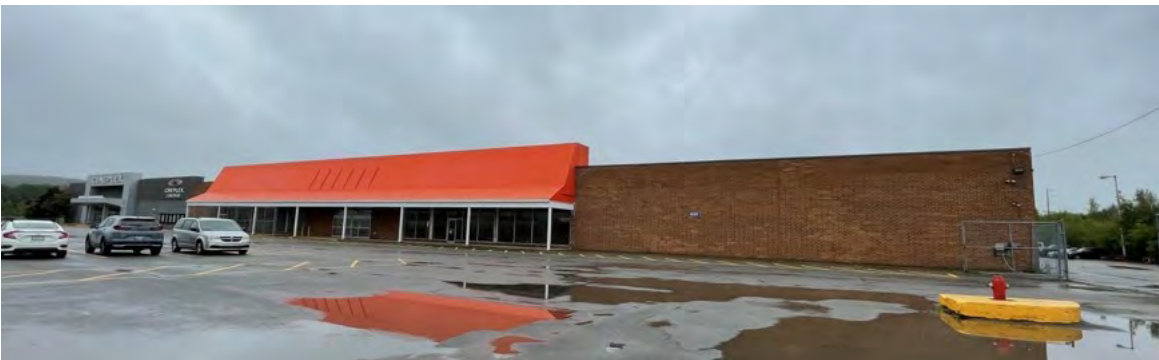
Figure 1: New Glasgow Transportation Department Facility front elevation.
