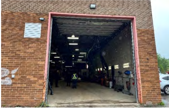
Figure 16 Side door providing natural ventilation
