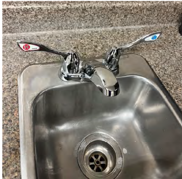
Figure 2 Typical Bathroom Fixture in Facility
