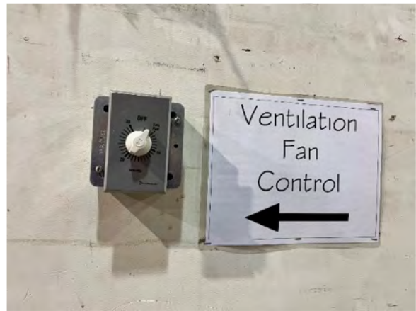
Figure 19 Exhaust Fan Control
