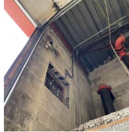
Figure 8: Opening in masonry wall.
