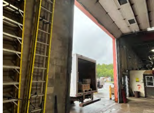
Figure 17 Back door providing natural ventilation
