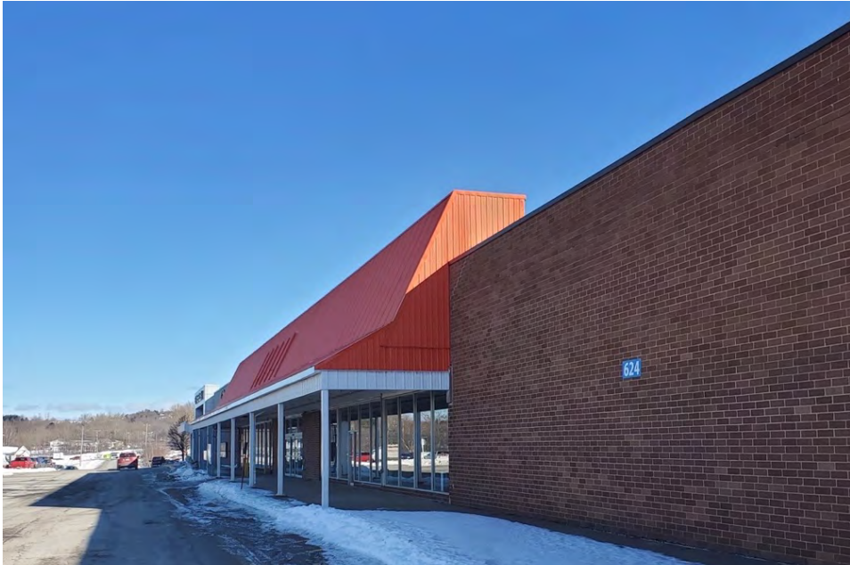
Figure 1 Municipal Operations Building
