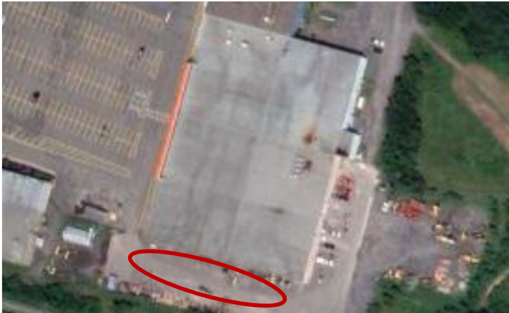
Figure 24 Location of Air Source Heat Pump
