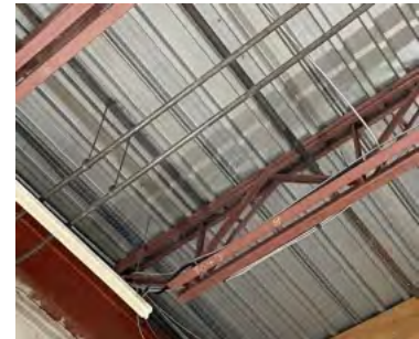
Figure 5: Open Web Steel Joist.
